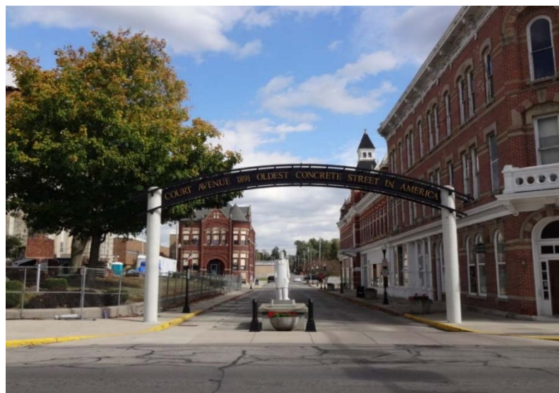
Figure 1.1 The oldest concrete street in America built in 1891 by George Bartholomew in Bellefontaine, Ohio (Image from www.trover.com ).
